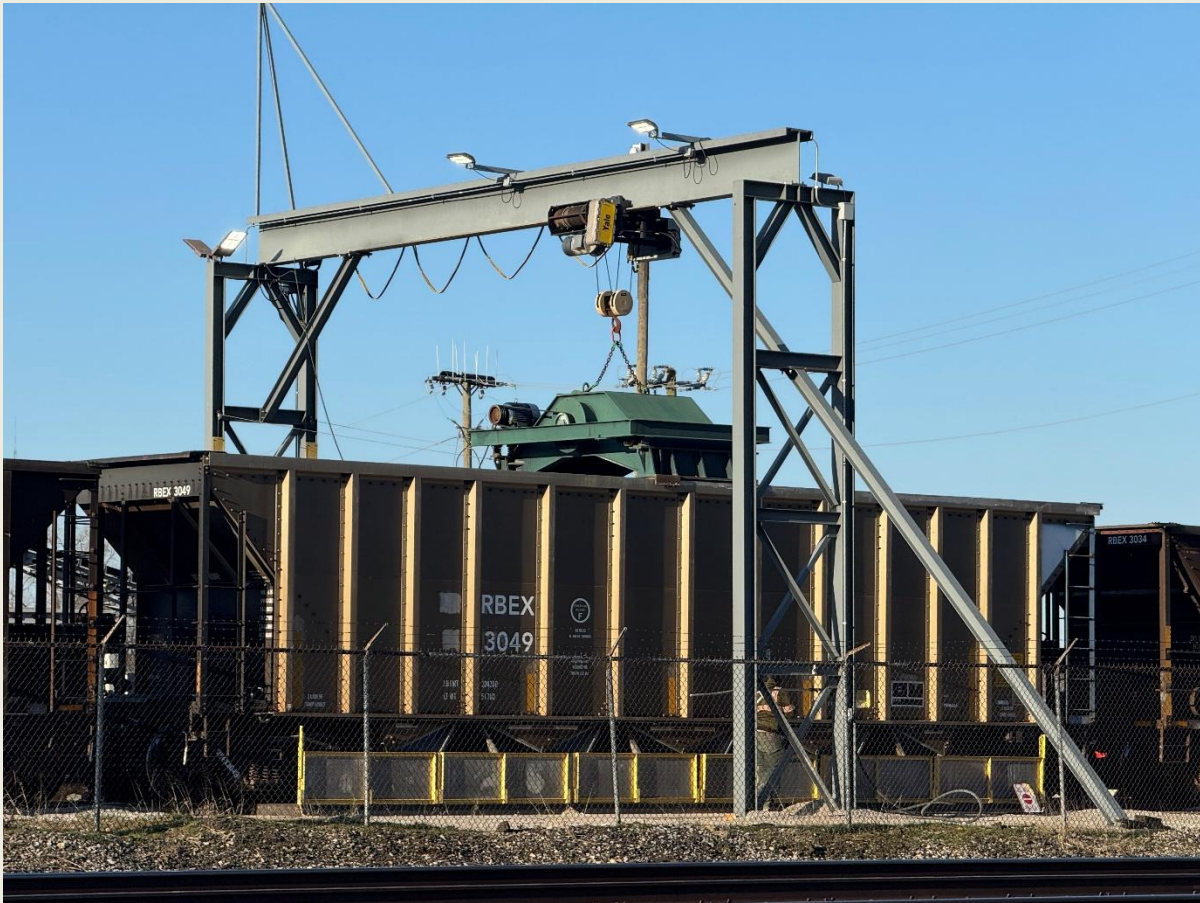
Car shaker at Balkama aggregate yard.
