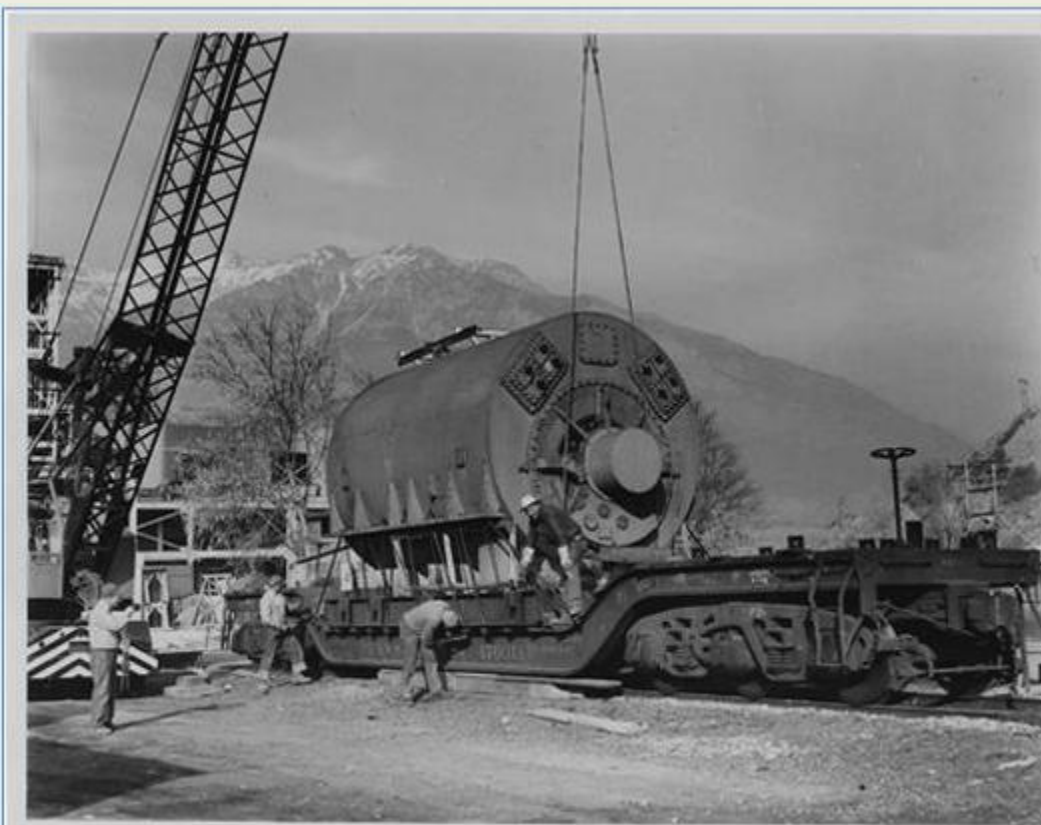
A Generator for a power plant
