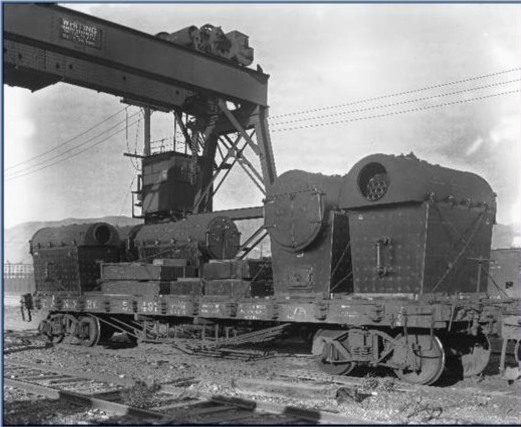
Stationary boilers on an all wood flat car
