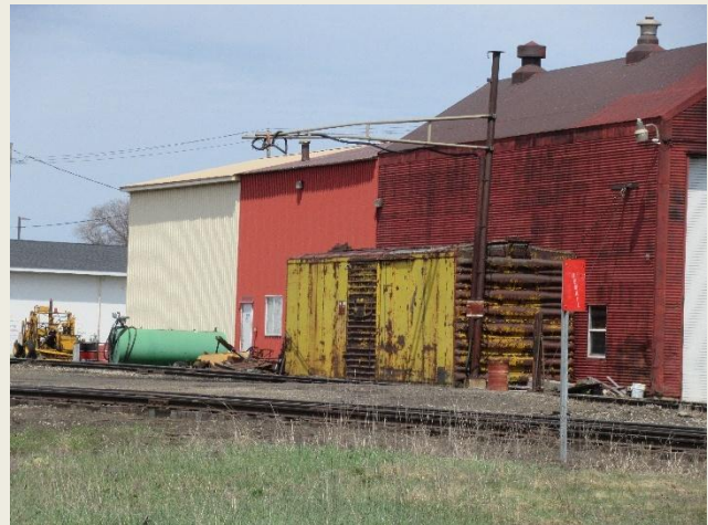
old box cars used for storage next to an engine house in Cadillac, MI
