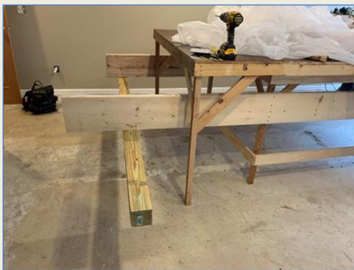
This picture shows some of the bracing that was added for additional support.
